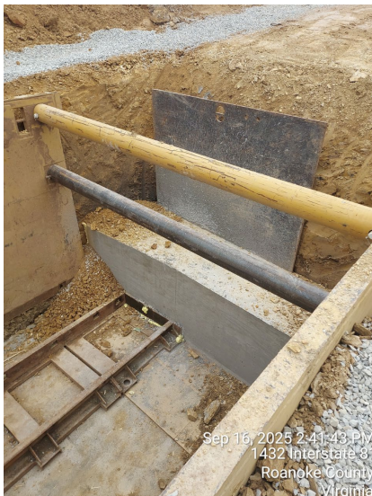
Boring Pit Assembly for the Wood Haven Technology Park Waterline Extension Project
