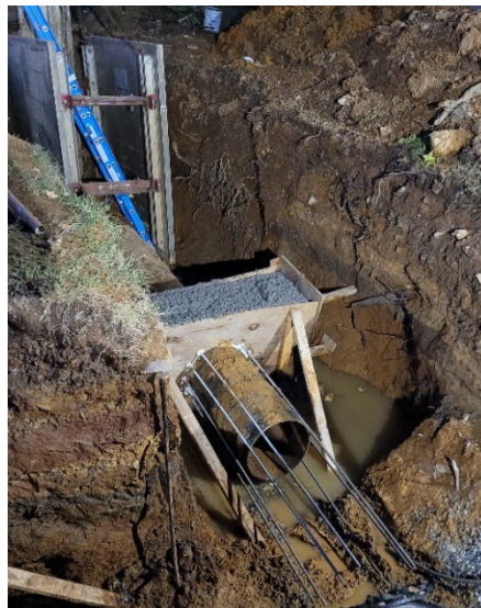
Pipe and fittings installed overnight by crews to get the 20-inch discharge main back in service at the Statesman Pump Station
