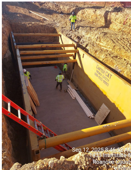
Boring Pit Assembly for the Wood Haven Technology Park Waterline Extension Project
