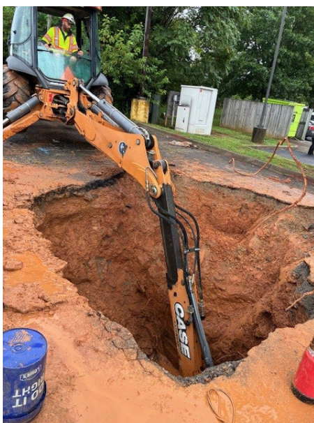
Excavating 15 feet deep to expose the break on the 20-inch transmission main
