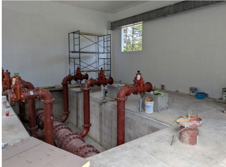
New 1385 Pump Station Structure with Roof Installed
